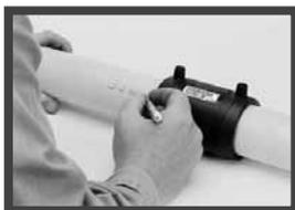
Fig. B8-1 : Mark fusion time on pipe Surface
